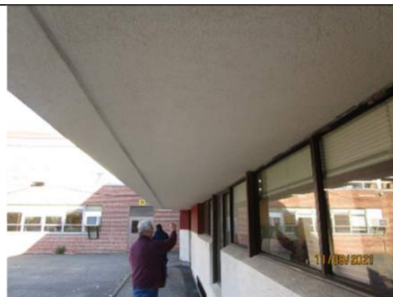
Little to no ventilation in the soffits.
