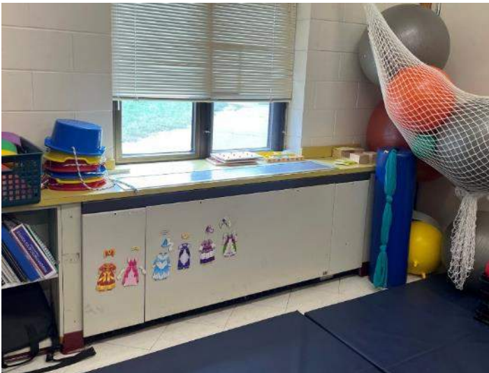
Figure 8: Unit ventilator with hot water heat and DX cooling original to the 200-Wing construction.
