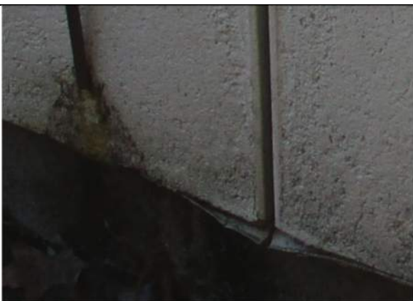
Ice damage at base trim and control joint.
