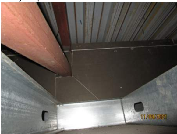
View inside the finish system soffit reveals that the gypsum sheathing on the exterior wall has no vapor barrier allowing drafts of outside air into the building.
