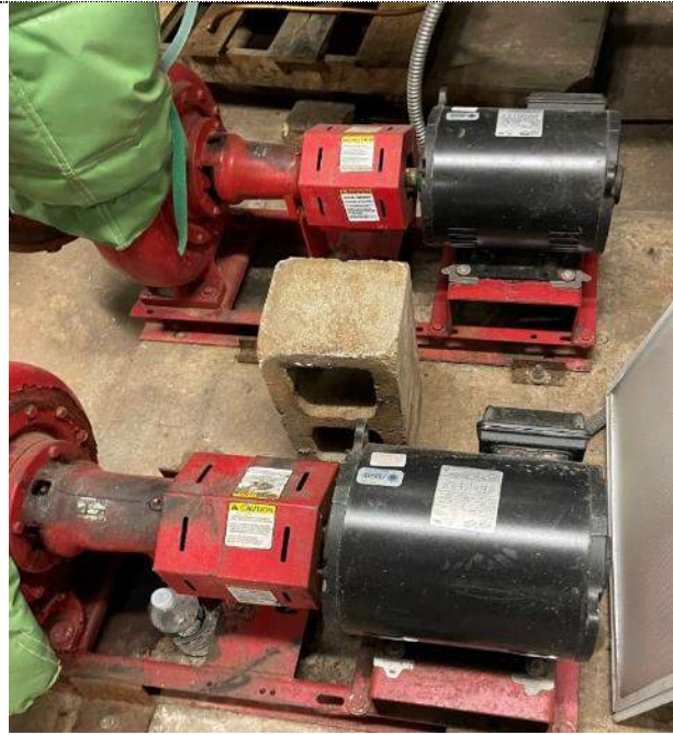
Figure 6: Heating HW pumps in boiler room
