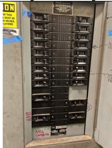
Figure 15: Old FPE panel serving the kitchen area
