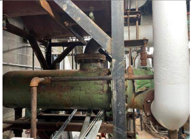
Figure 4: Steam to hot water HX in the boiler room
