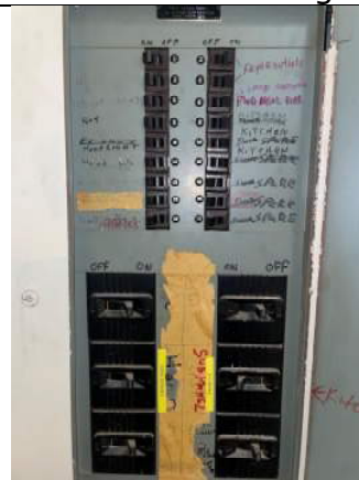
Figure 18: Old FPE panel outside the boiler room
