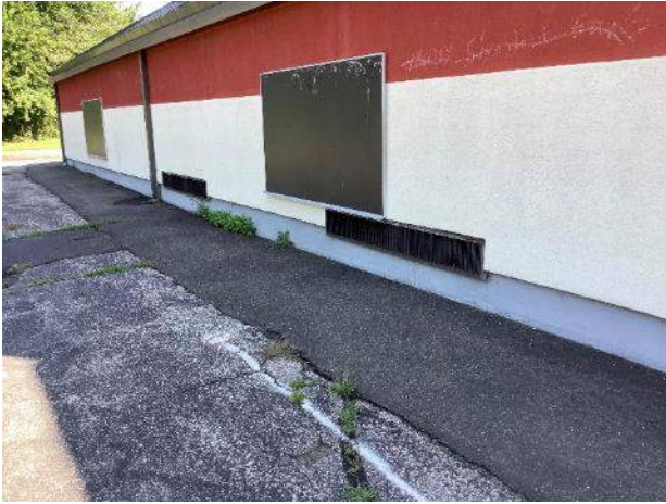
OA grills on the outside wall for fan coil unit ventilation.
