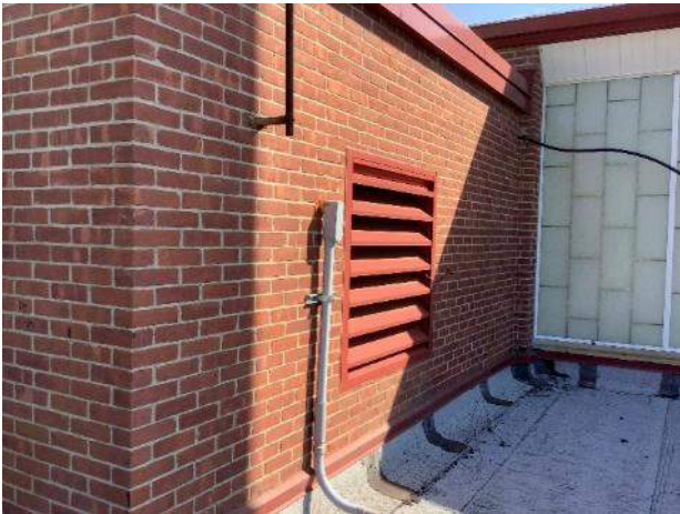
OA louvers on the exterior of wall of the building as observed from the roof.
