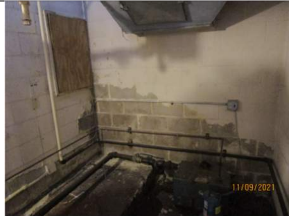
Evidence of hydraulic water pressure against the below grade wall and water infiltration into the building.
