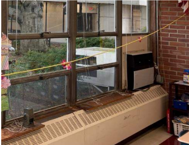
Figure 7: Steam radiation and window AC unit in the original building
