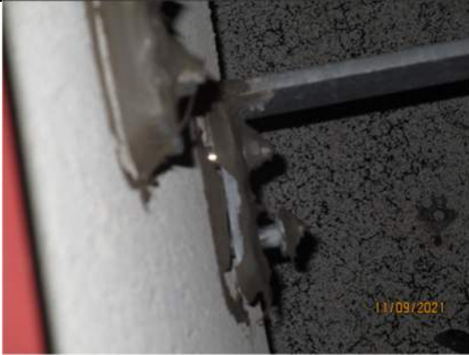
Roof ladder pulling away from the building causing the sealant around the anchors to tear allowing water into the wall.
