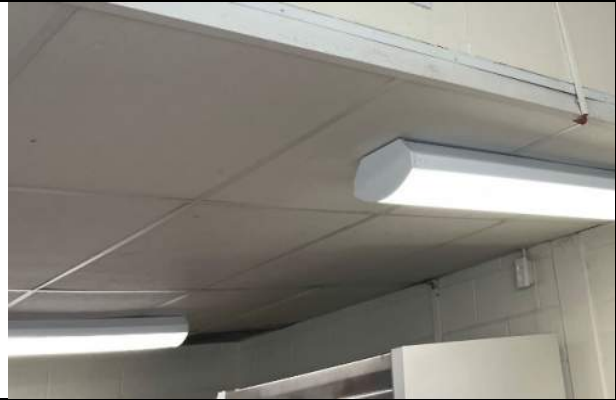
Figure 24: Surface mount LED fixtures in kitchen
