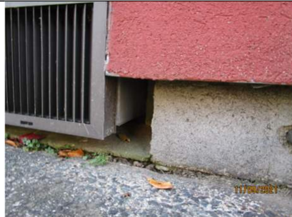
Wide open-air gap at the unit ventilator into the building.
