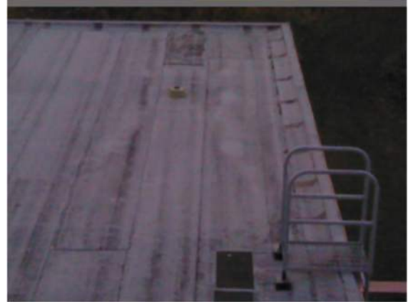
Thermal pattern consistent with water infiltration at the roof ladder possibly caused by the movement of the ladder due to the loose anchors.
