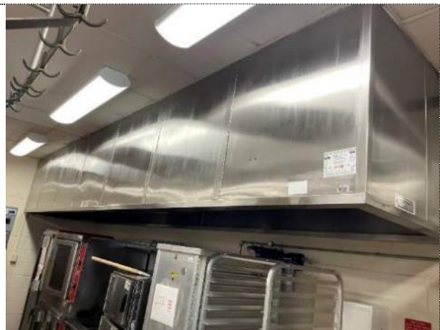
Figure 11: Kitchen exhaust hood.
