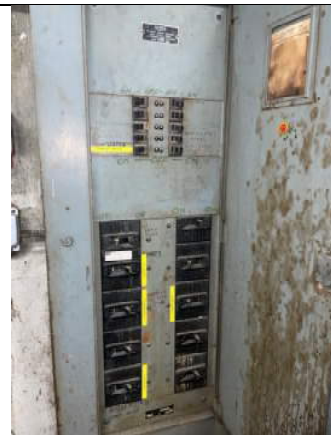
Figure 17: Old FPE panel serving boiler room
