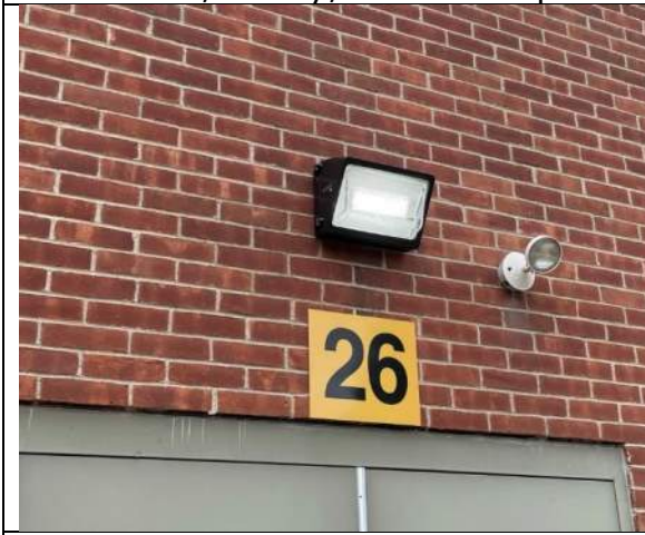
Figure 25: Exterior LED WallPak fixture
