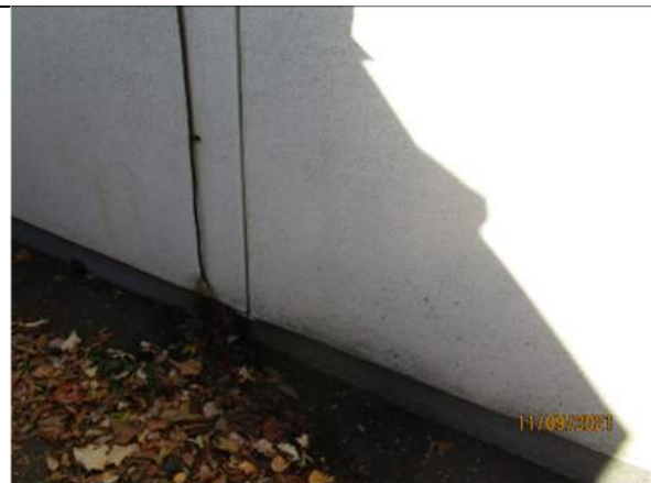
All the base trim and control joints appear to have expansion damage from water exfiltrating the system and expanding when leaving the system.
