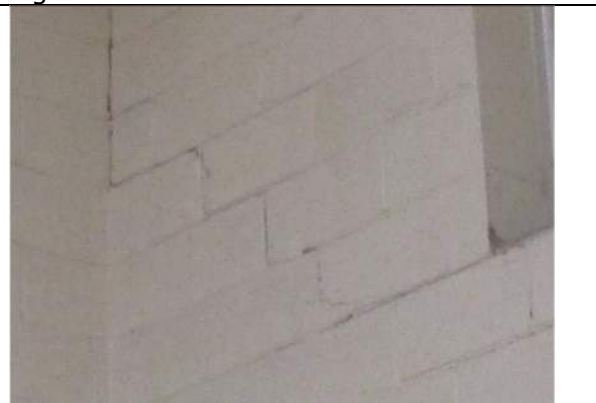
Cracking continues to the opening.
