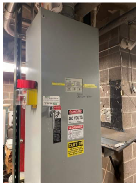
Figure 22: New 400amp ASCO Automatic Transfer Switch
