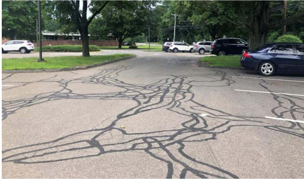
Cracking along pavement. Future pavement repair 5+ years.
