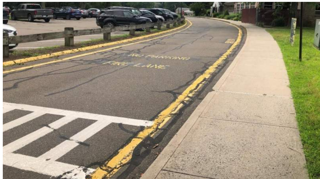
Cracking along pavement. Future pavement repair 5+ years with re-stripping.
